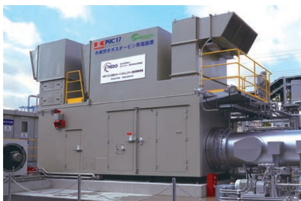
Fig. 10 Cogeneration facility with flexibility in the fuel mixing ratio of hydrogen to natural gas
