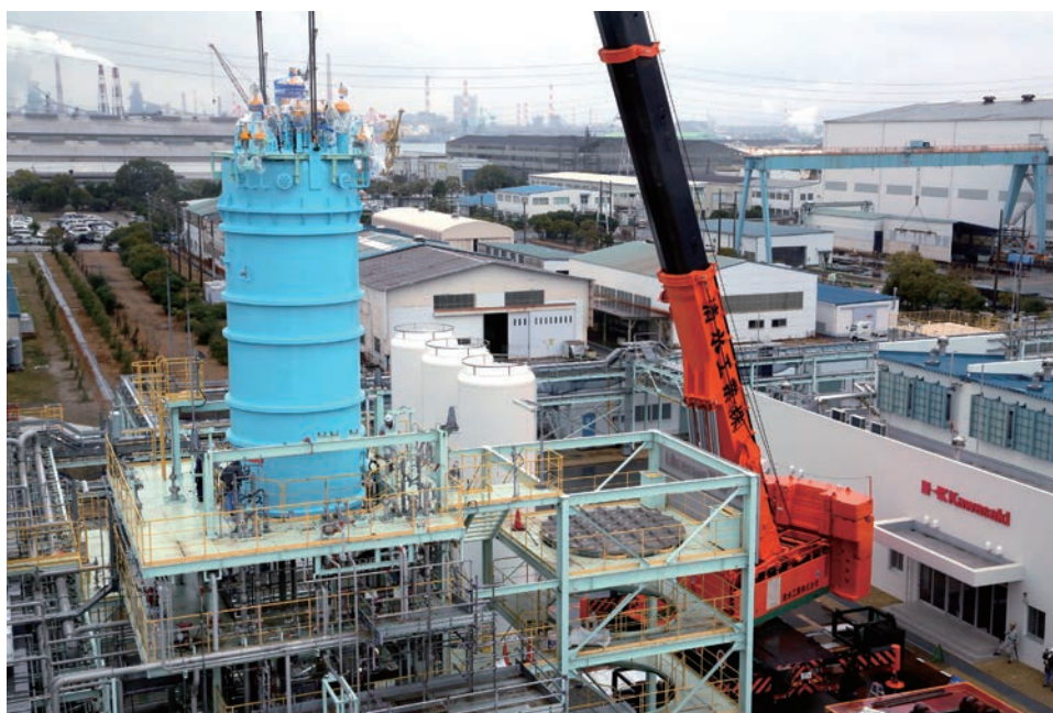
Fig. 5 Installation of new liquefier
