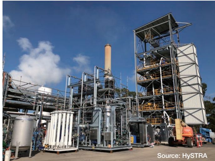
Fig. 6 Brown-coal gasification and hydrogen refining facility (February 2020)
