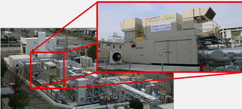
Figure 2: World’s first pure hydrogen and natural gas demonstration plant in Kobe (Japan)
